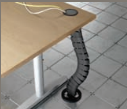
Cable snake : direct access to floor services
